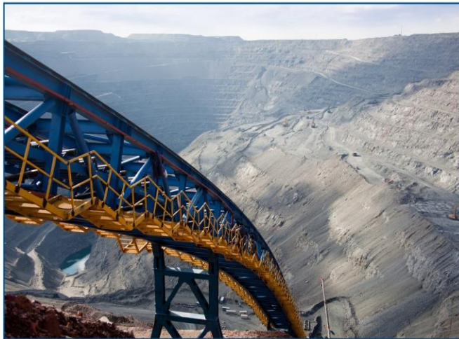
Overland Mining Conveyor- Typically the conveyor drives and tension roll bearings are the components monitored. When one drive on this conveyor is down the whole mining operation is down.
